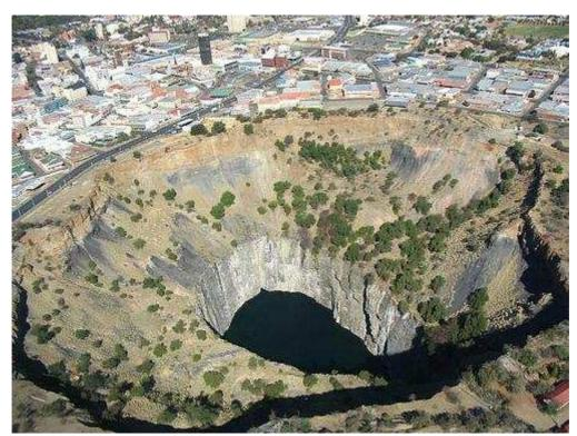
Apparently the largest ever hand-dug excavation in the world, this 1097 meter deep mine yielded over 3 tons of diamonds before being closed.
