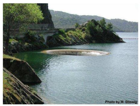
A glory hole is used when a dam is at full capacity and water needs to be drained from the reservoir.
