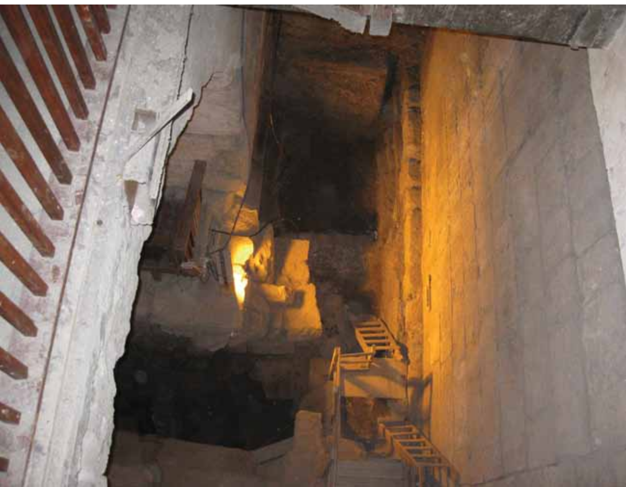
Excavation in The Western Wall's Tunnel - 2011
