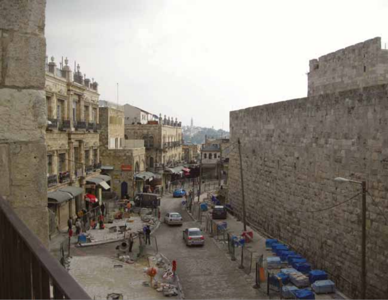
Construction works near Jaffa gate
