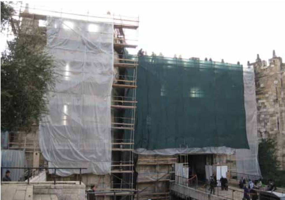
Damascus Gate/Bab Al-Amud preservation work 2011
