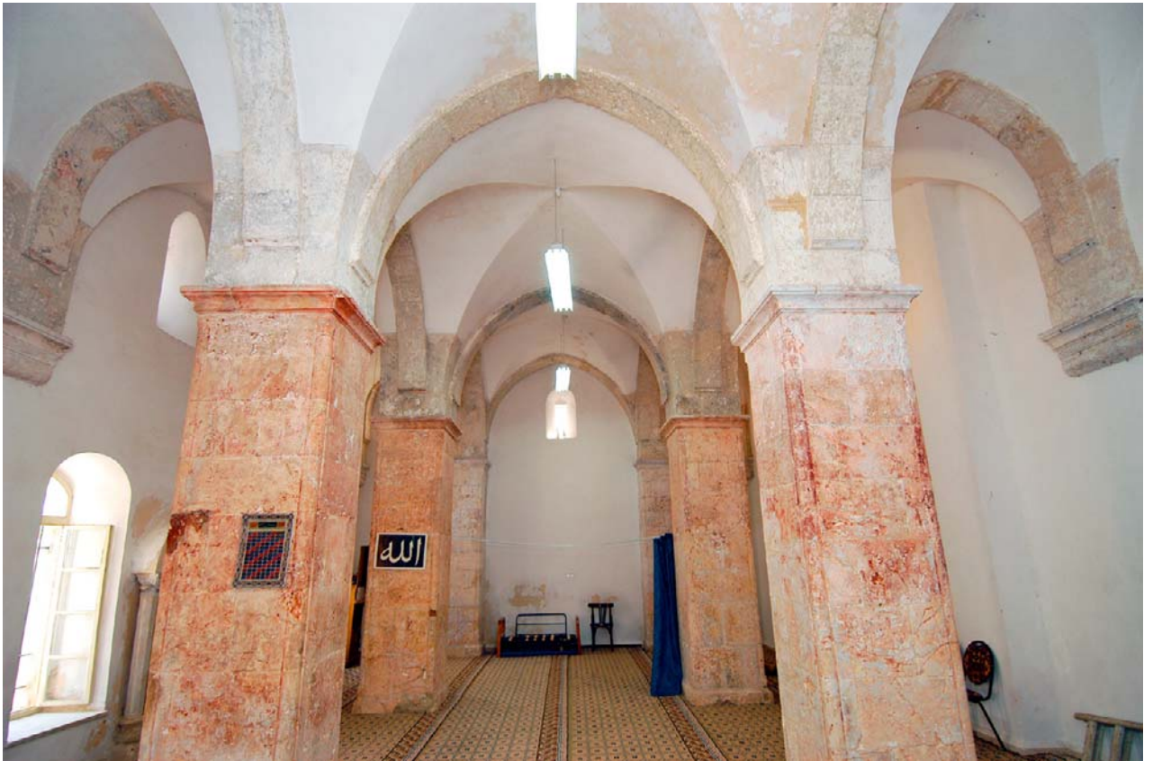
In al-Malawiyya Mosque, previously unknown spaces below ground level were discovered, restored and utilized.
