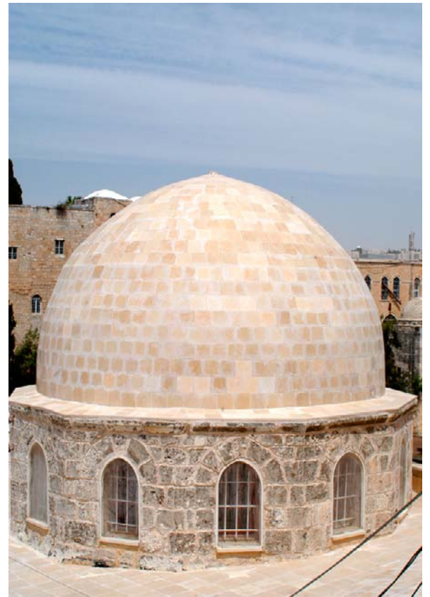
Insulation and tiling of the dome and roof of Al-Madrasa al-Manjakkiya was completed in 2003.
