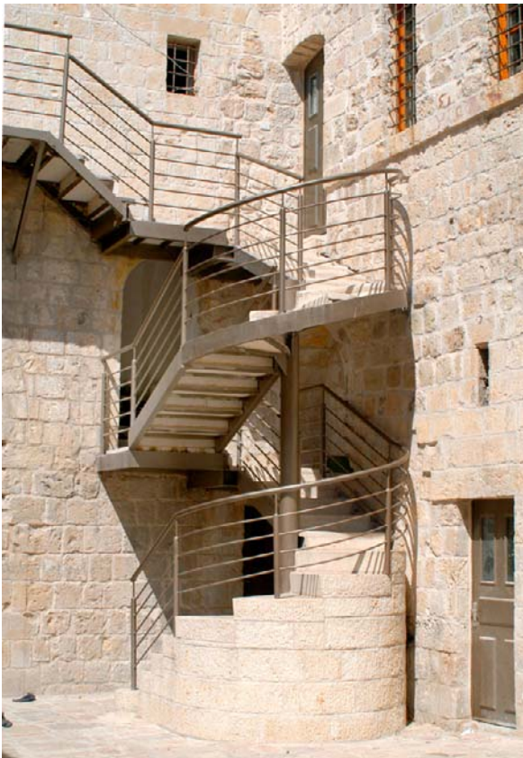
The industrial training school. All new additions to the old structures are of a reversible nature.
